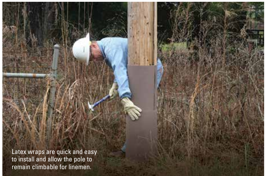
Latex coatings and wraps allow the pole to withstand multiple burns making it more cost-effective for pole owners.
